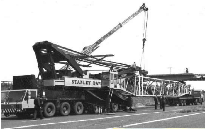
Left - Colossus being setup for a heavy bridge lift on motorway construction. Although supposed to be self erecting this is obviously using a second crane for assembly
