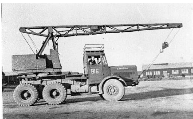
Below Left - EMA fitted to an AEC Matador Lorry chassis.
