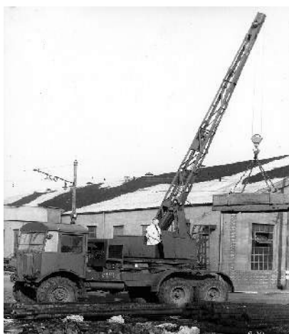
Below Left - EMA fitted to an AEC Matador Lorry chassis.
