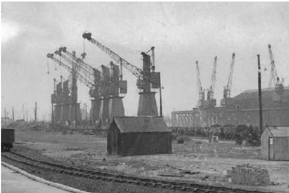
Above - water hydraulic 30Ton 66.ft lift 1915.
