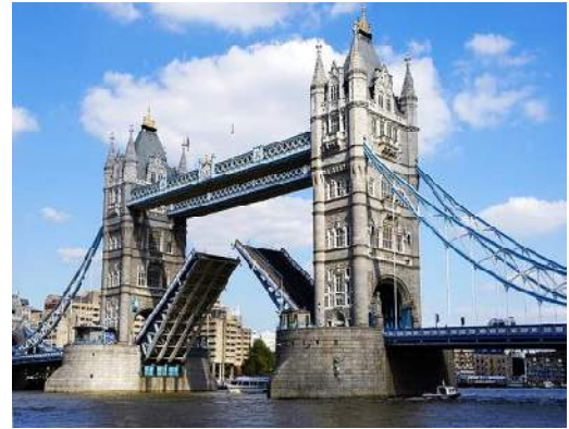
Right - Tower bridge built in 1894 used water power to raise the bridge sections.
